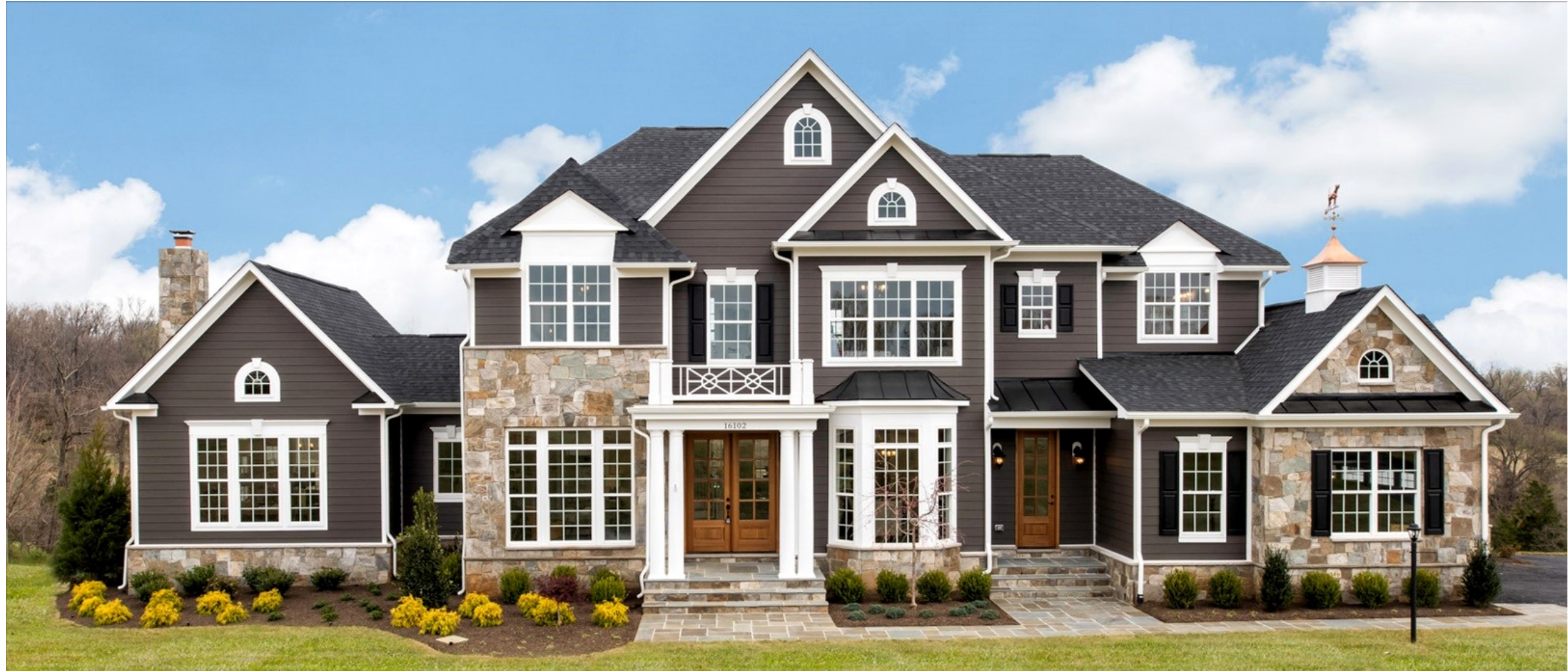
Elevation 7A shown with optional stone, mahogany doors, service entrance, and side club room
